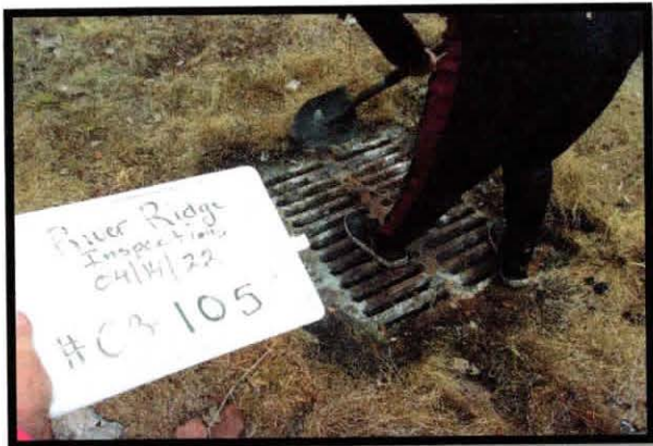
Could not inspect because grates were falling apart when we tried to lift up. Recommend new grates
