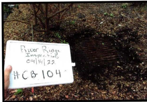
Could not inspect because grates were falling apart when we tried to lift up. Recommend new grates
