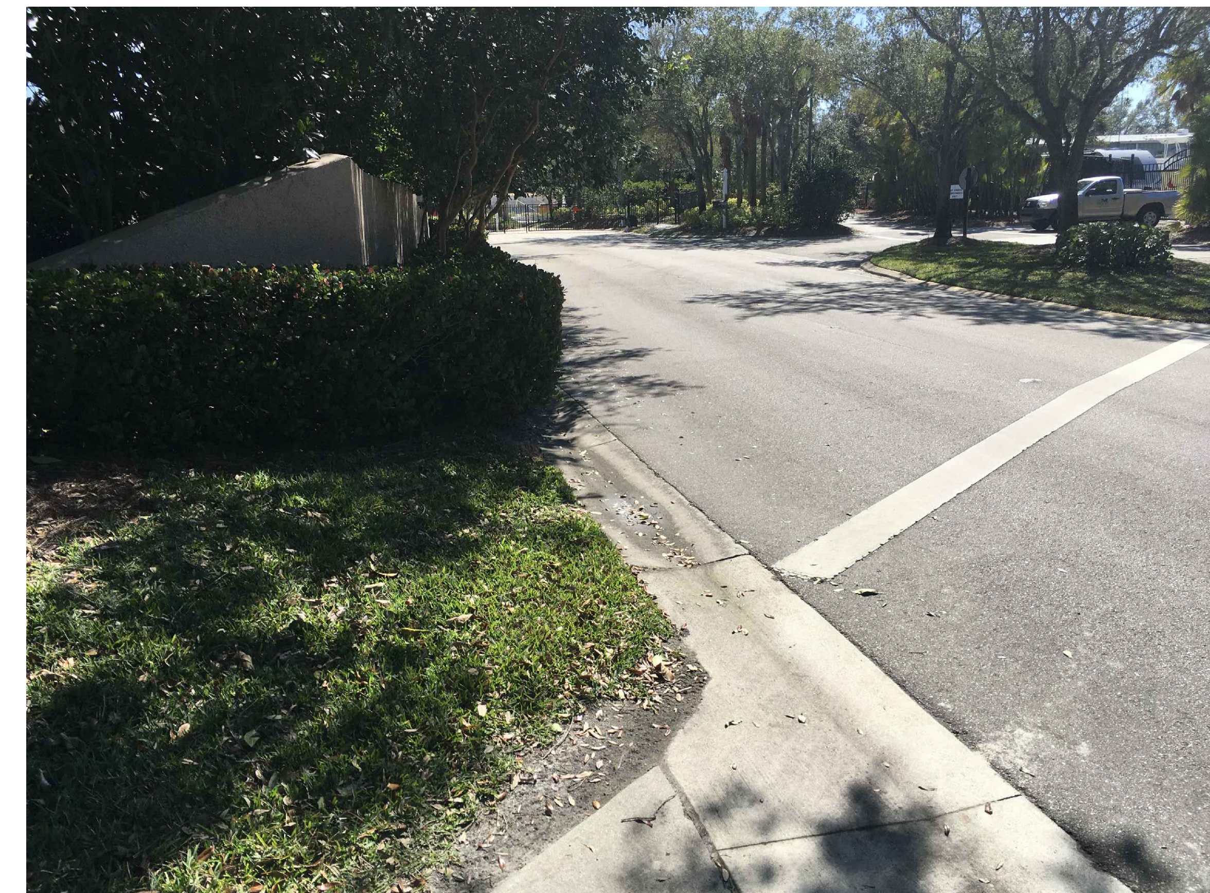
GOLF CART CROSSING (SOUTHEAST SIGHT LINE VIEW)
