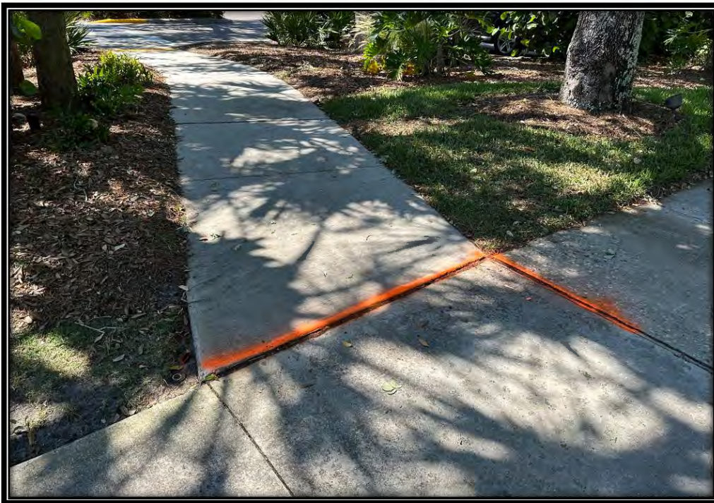
Figure 3: Raised sidewalk along Pelican Sound BLVD in front of west parking lot of Clubhouse.
