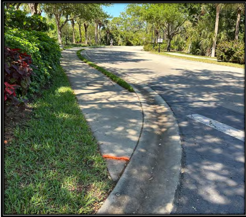
Figure 2: Raised sidewalk at intersection of Island Sound Cir and Hammock Greens Ln.
