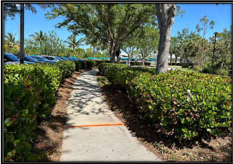
Figure 1: Raised sidewalk along Pelican Sound BLVD near pool area along first parking lot.
