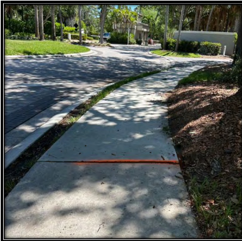
Figure 7: Raised sidewalk transition approaching roundabout and community entrance/exit on Pelican Sound BLVD.
